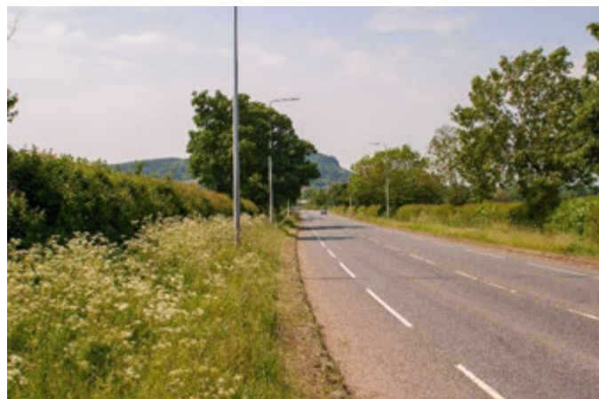
A56 looking toward Helsby High School with cycle-lane and broad grass berm.
