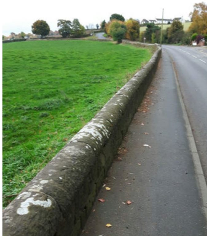
The footway from Lady Heyes to Kingsley; Shared Use paths less than 3m width are an exception normally only permitted for short stretches. (DfT guidelines, see 1.3)
