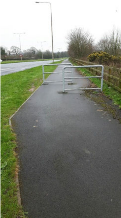
1.4 Shared use scheme in the rural environment; a wide well surfaced path separated from the roadway. (Daresbury, Cheshire)
