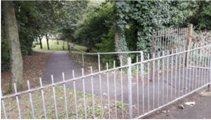
Looking down FP59 toward the Station Car Park; inadequate lighting dis-incentivises all users.
