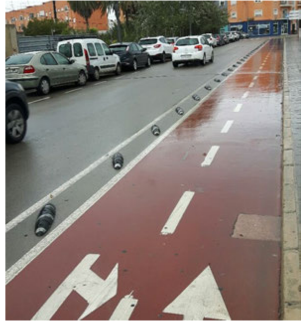
1.5 Segregated infrastructure in the urban environment; 'armadillos' remind motorists if they leave the carriageway! (Denia, Spain)
