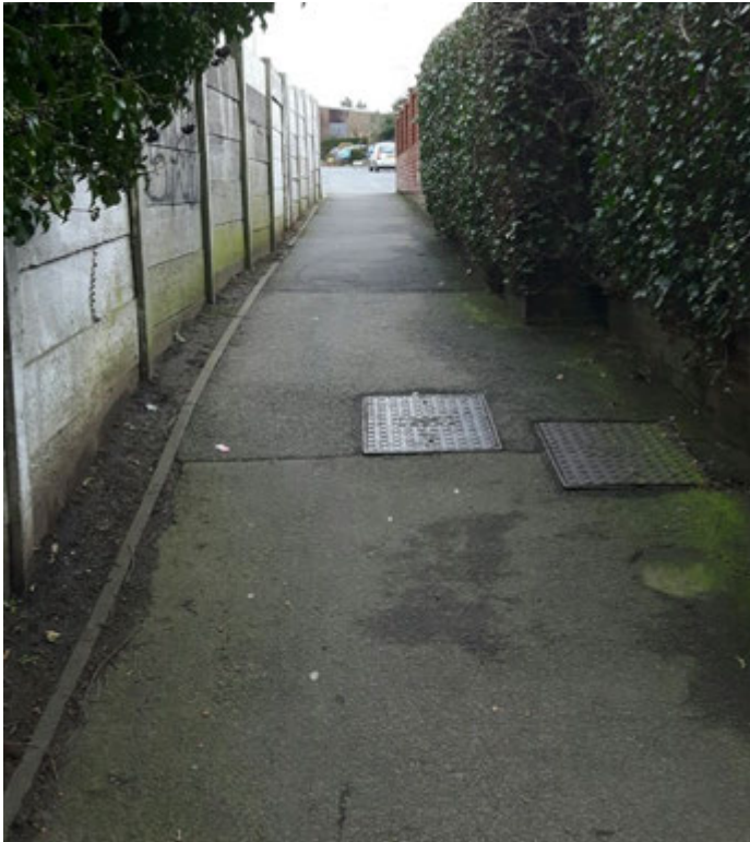
The narrow alley connecting FP56 and the London Rd path with Blue Hatch; not suitable for shared use and cyclists should dismount. Signage would be needed.
