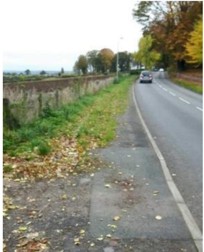
The footway discontinuity along the B5152 looking toward Kingsley; the need for several crossing points and encroached surface makes the footway unsuitable for Shared Use.
